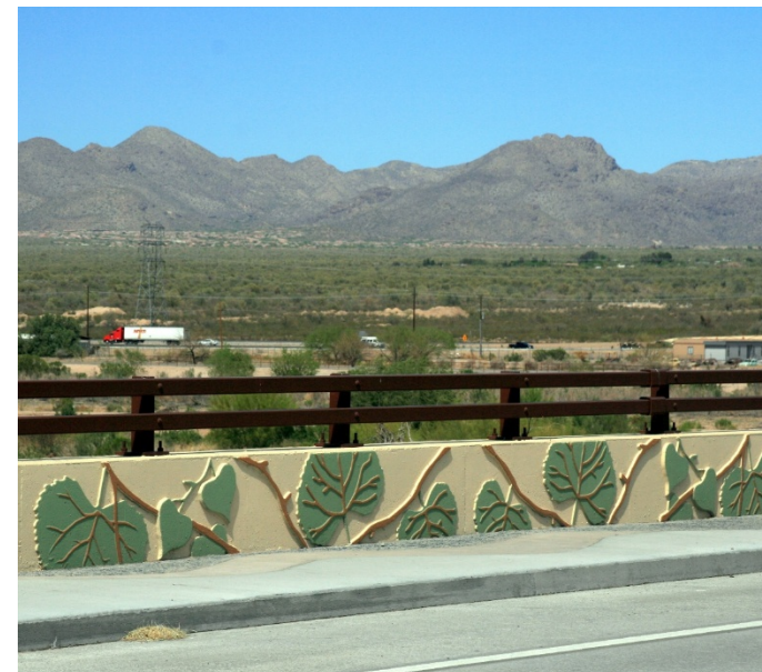
Bridge Barrier Formliner
