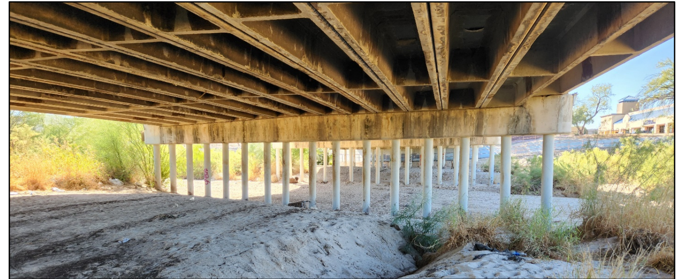
Figure 14 - View of Existing Bridge Pier, Piles, and Underside of Girders
