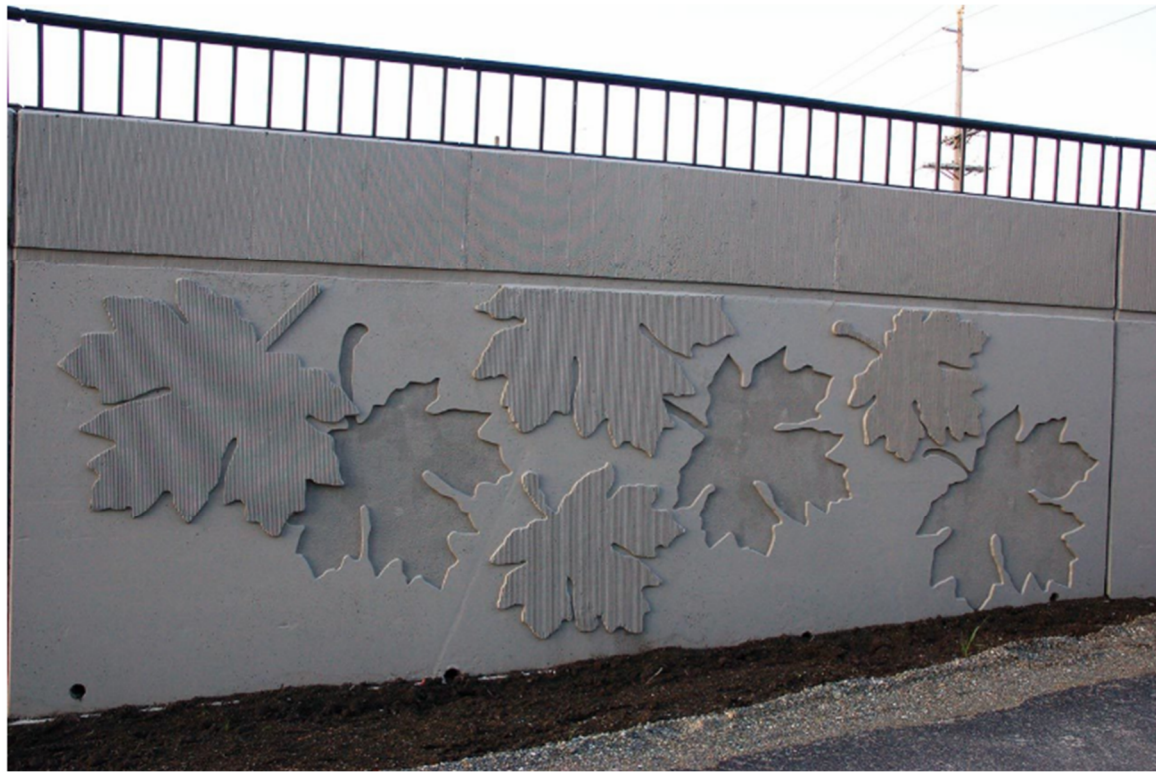
Retaining Wall Formliner
