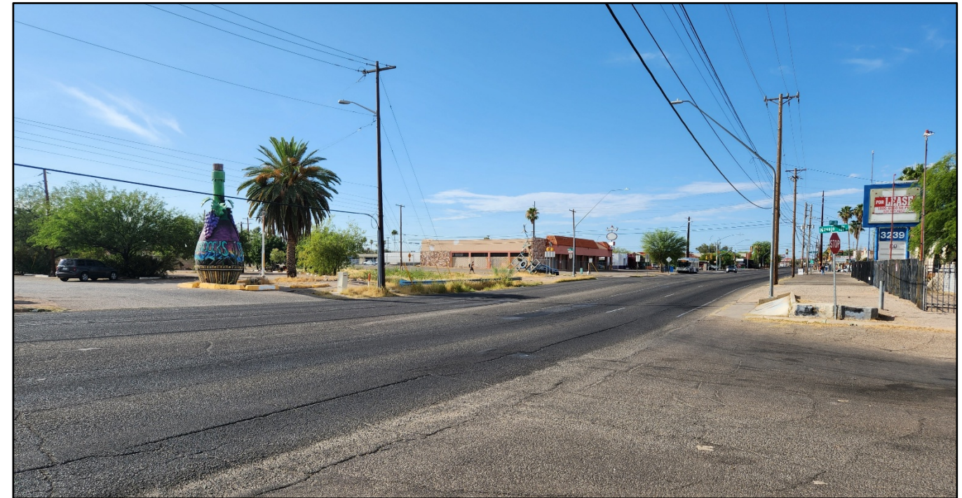
Figure 11 - Navajo Wash Dip Crossing 1 st Avenue (Looking South)
