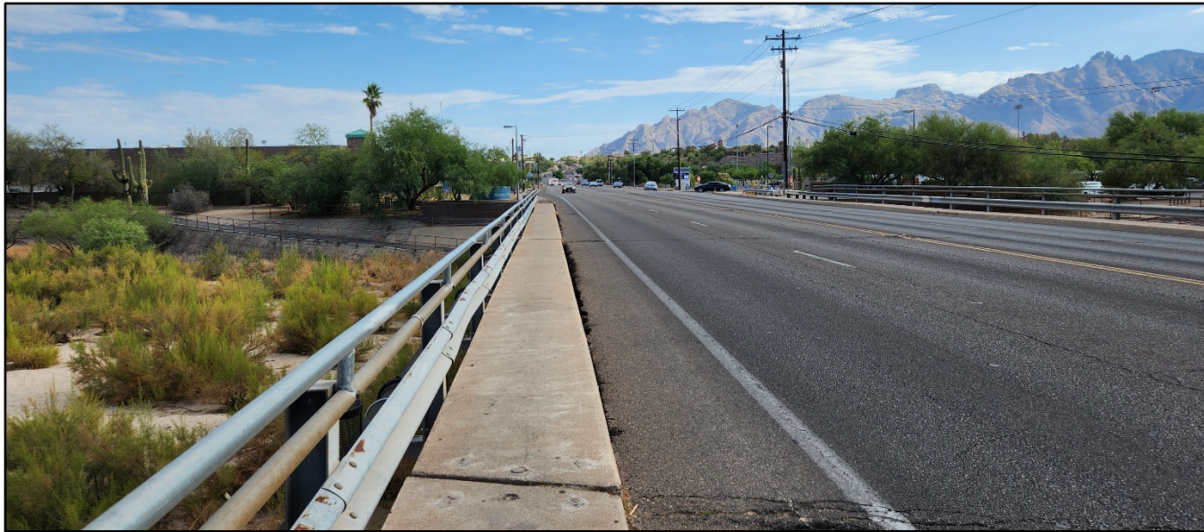
Figure 12 - Existing Bridge Railing, Sidewalk and Drainage (Looking North)
